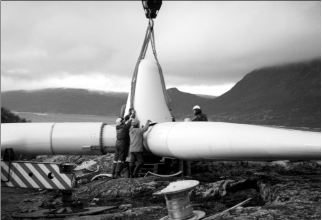
Preparing to raise the blade assembly into position.
